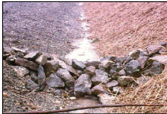
Rock check dams slow down stormwater in swales, reducing erosion
