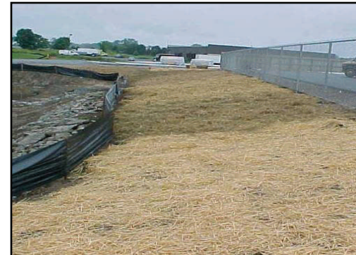
Construction Site Stabilized with Straw Mulch
