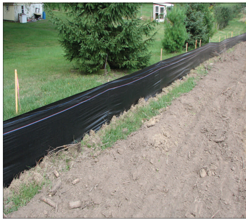
Properly installed and maintained silt fence.
