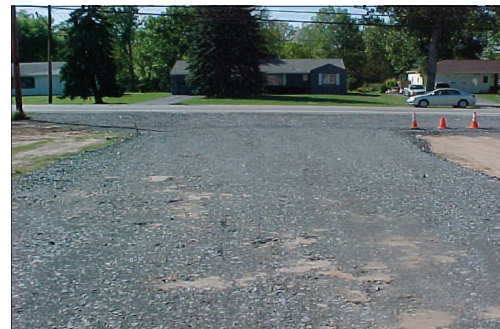
Properly installed construction site entrance.
